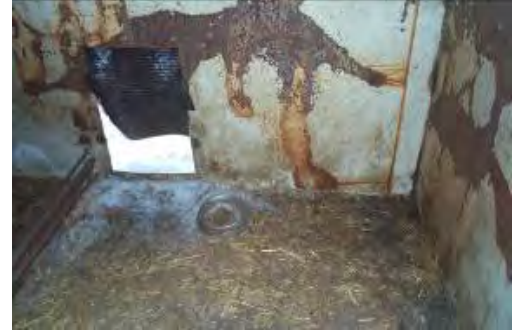
8-21. No bedding, rusted dog enclosure 3.1(c)(1)(i); 3.3(a)
